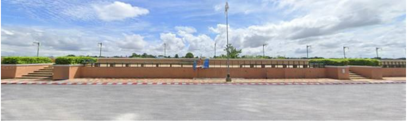
Current Floodwall and Riverbank Barrier along the Chao Phraya River in Singburi Province The existing structure is a permanent concrete flood barrier that helps prevent flooding but obstructs the view and limits access to the riverbank.
